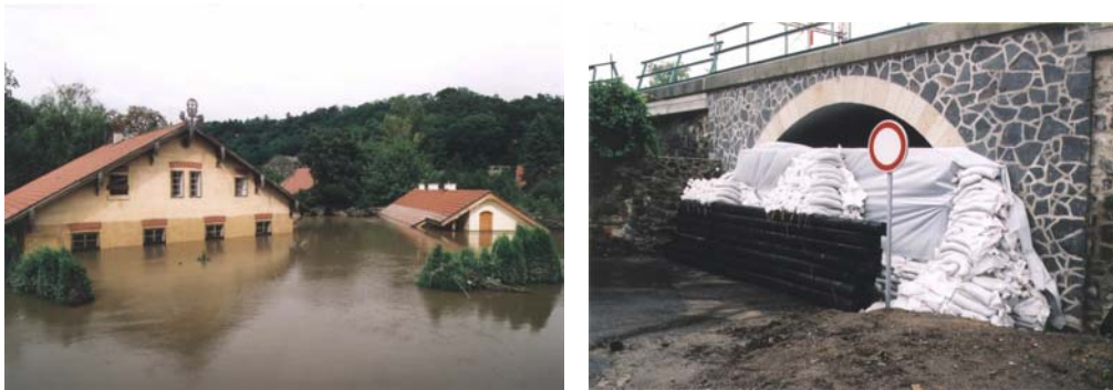
Flooded building with plasmochemical reduction and roadblock
